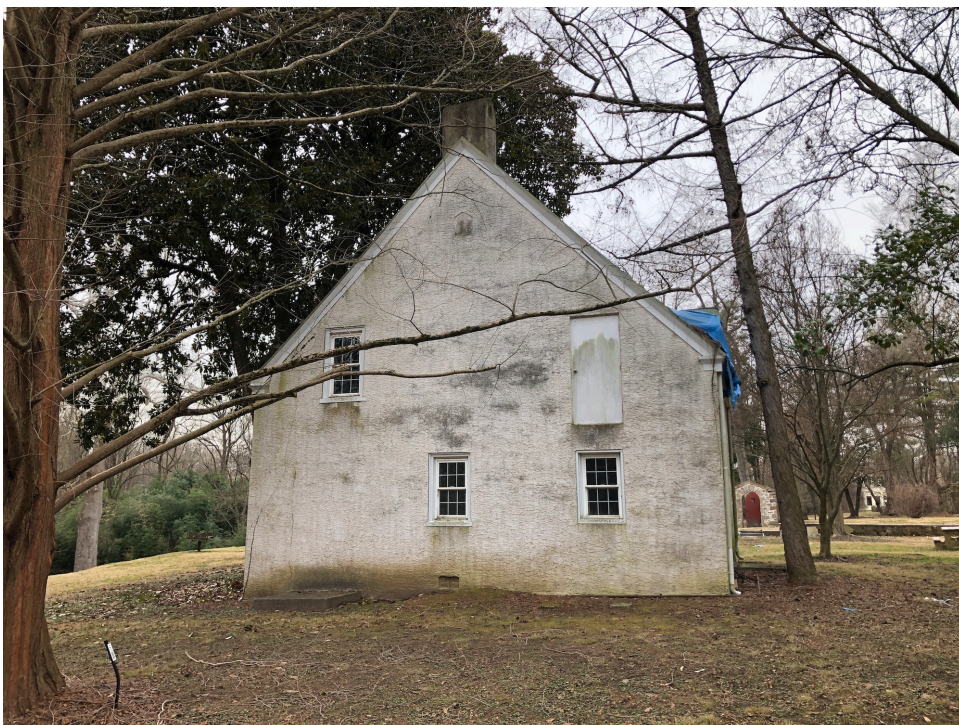
Fig. 10. Chimney of the 1946 addition. Current photo.
