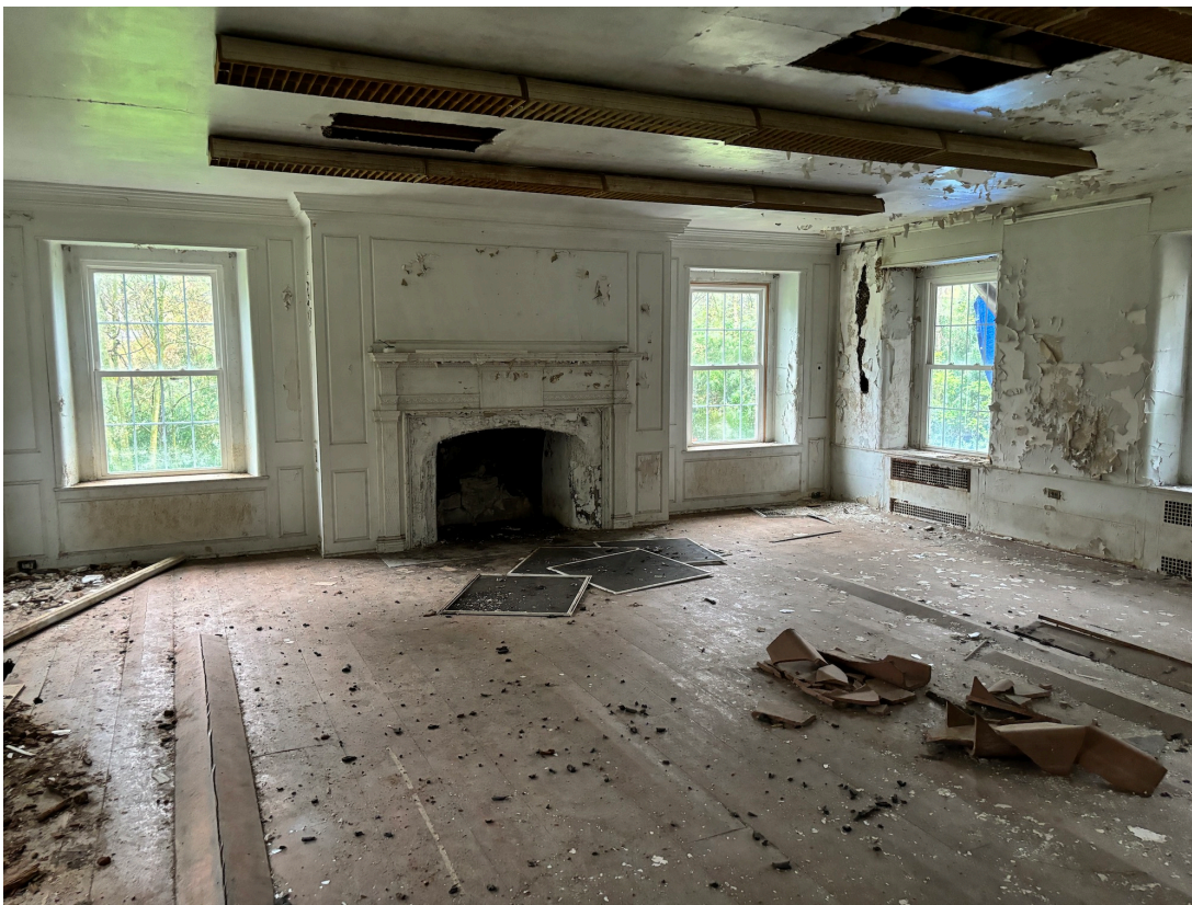
Fig. 19. Large fireplace and windows downstairs in the 1932 addition Current photo.
