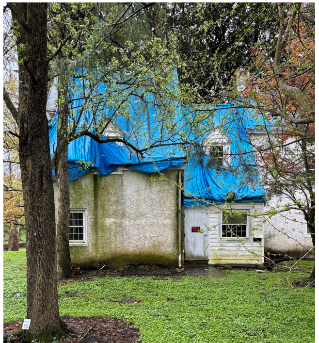
Fig. 14. The north face of the servants quarters as actually built with later stucco on mesh added and door changed. Current photo.
