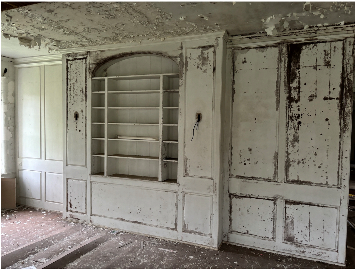
Fig. 29. Built-in shelving upstairs in the 1932 addition. Current photo.
