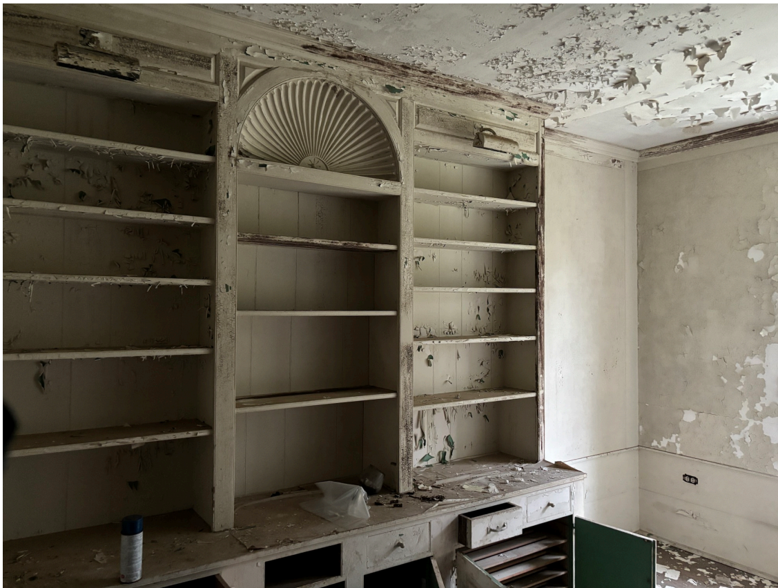
Fig. 24. Built-in shelving downstairs in the 1932 addition Current photo.
