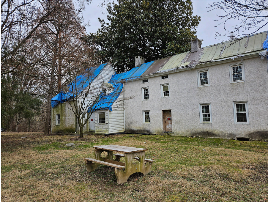
Fig. 7. Clapboard siding on part of the 1946 addition on the left in the photo. Current photo.
