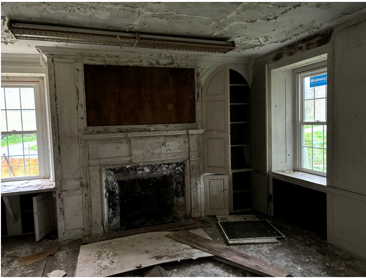
Fig. 25. Built-in cupboards next to the fireplace at the west end of the c. 1820 portion of the house. Current photo.
