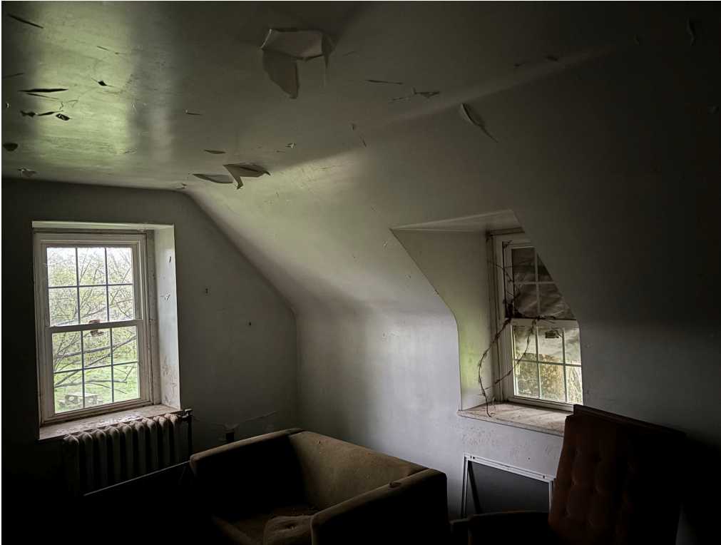
Fig. 31. Arched ceiling with curved corners upstairs in the 1946 addition. Current photo.
