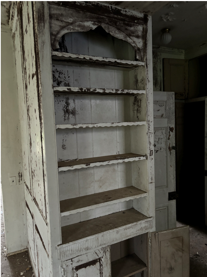
Fig. 28. Built-in shelving and cupboards downstairs in the 1932 addition. Current photo.
