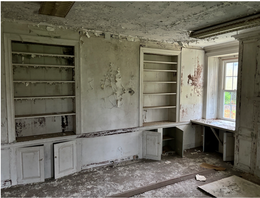
Fig. 27. Built-in shelving and cupboards downstairs in the 1932 addition. Current photo.
