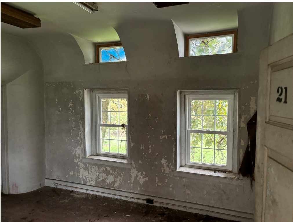
Fig. 32. Curved ceilings around the eyebrow windows upstairs in the c. 1810 portion of the house. Current photo.
