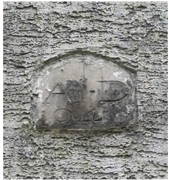
Fig. 41. The date stone as it currently appears, surrounded by rough stucco that was added much later.. Current photo.
