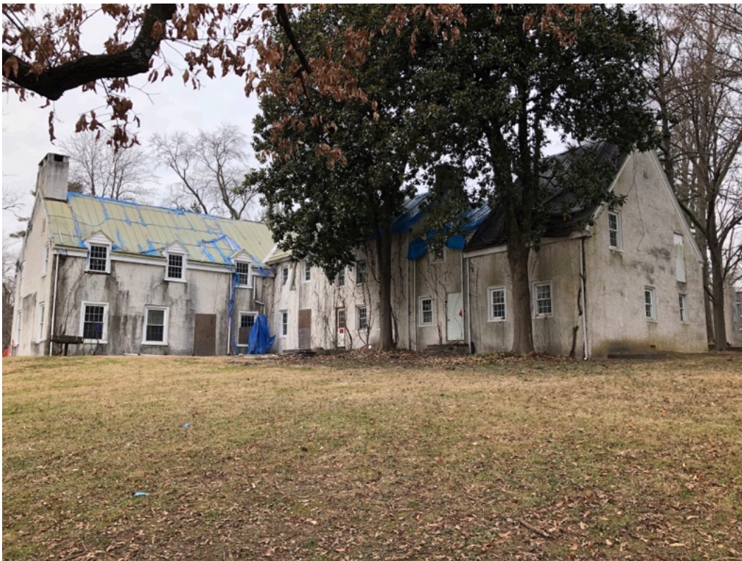
Fig. 35. The south and east side of the house, looking northwest. On the right is the 1946 east side addition to the servants quarters. Current photo.
