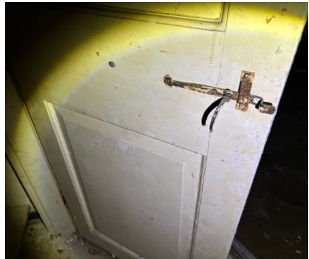
Fig. 43. Antique door latch in the servants quarters upstairs. From the archives of the King of Prussia Historical Society..
