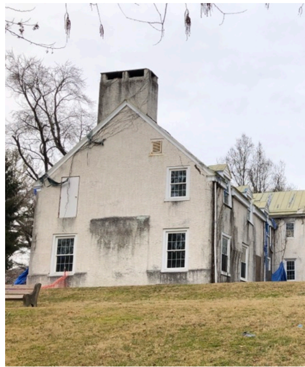
Fig. 48. The south side of the 1932 Okie addition, showing the emergency exit from the second floor. Current photo.
