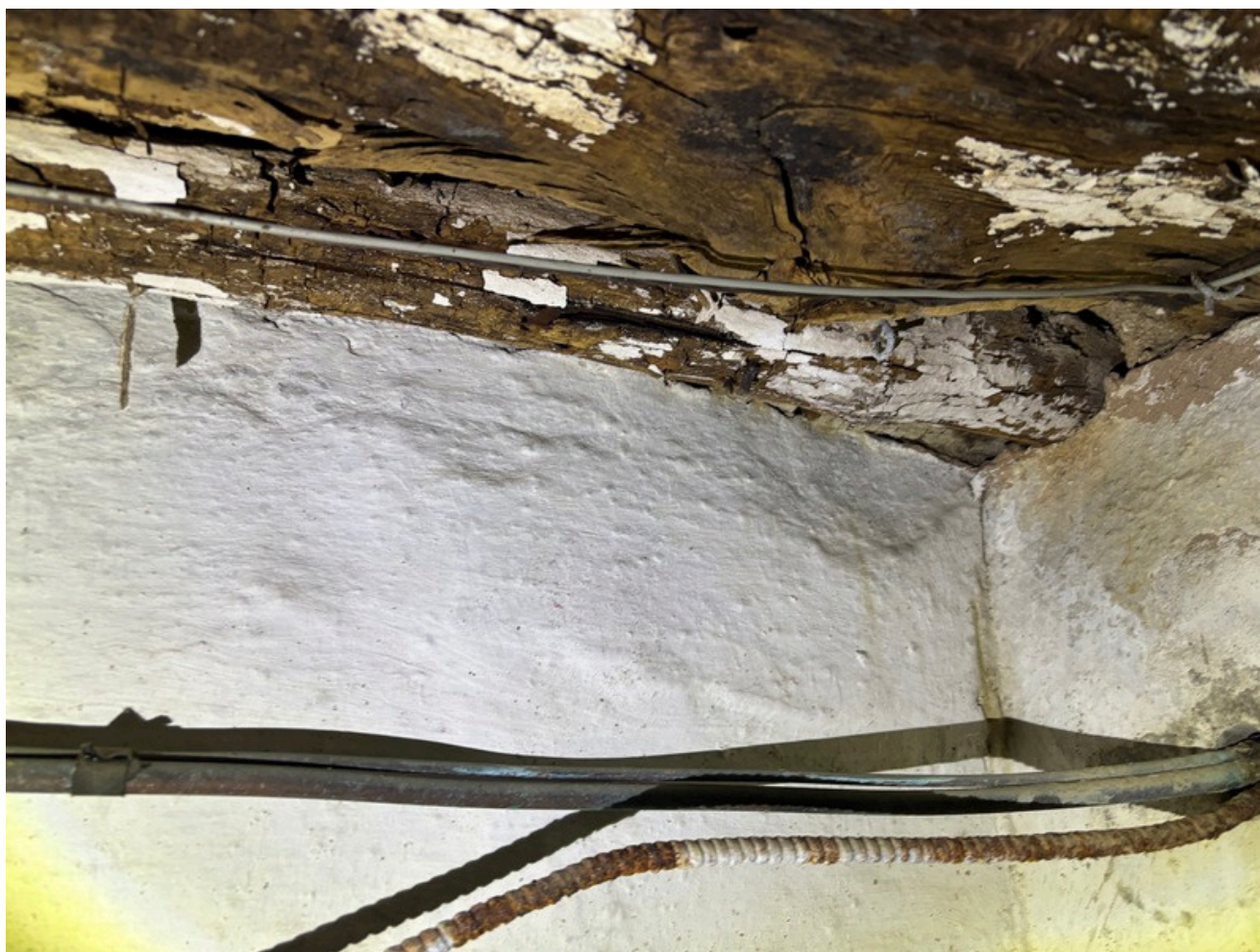
Fig. 14. Rough wood in the fireplace wall, as seen in the basement. King of Prussia Historical Society.
