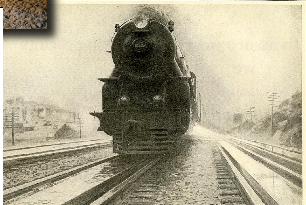
The locomotives of the Pennsylvania Railroad take water on the fly from long tanks between the tracks.
