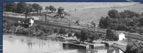
1940 - North Abrams Tower & Water Tank - Catfish Lock & Dam - PHMC - PA State Archives - MG-416-1 21089
