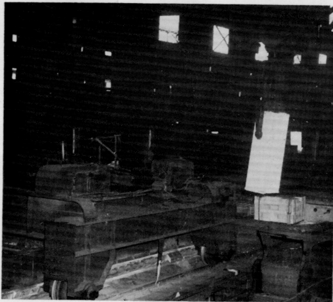
Ingot from Open Hearth Department goes into Blooming Mill "soaking pit."
