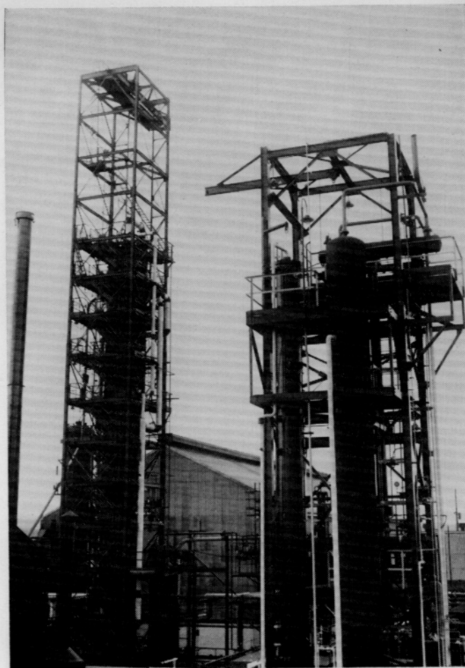
View of the Hydrogen Production equipment is shown in the foreground, with the reducer tower to the left. Finishing building is in the background.
