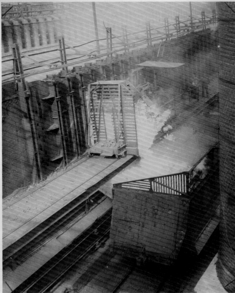
Quenching car receiving a load of hot coke, which is being pushed from an oven.
